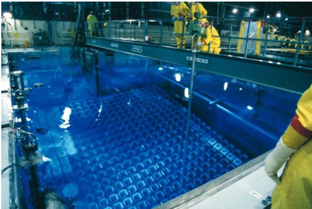
Used nuclear fuel is stored at least 20 feet below the water's surface.
